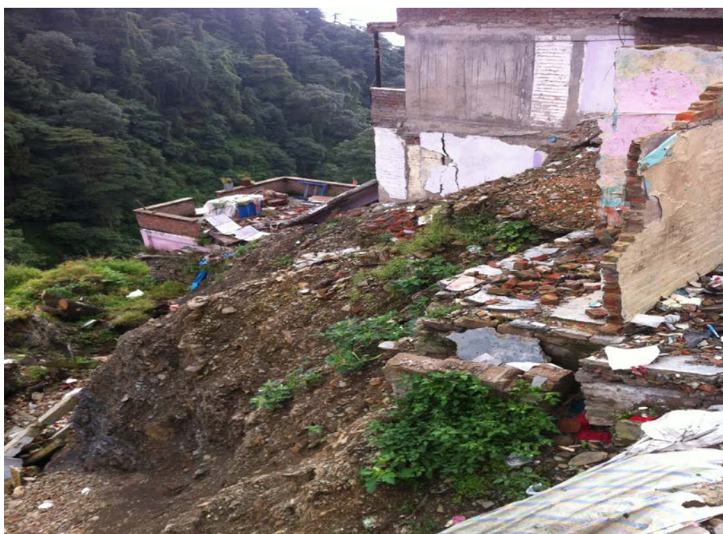
Figure 2: Houses in the Krisna Nagar slum were devastated by landslides in 2012 and 2013 © Helen Scott 2013
