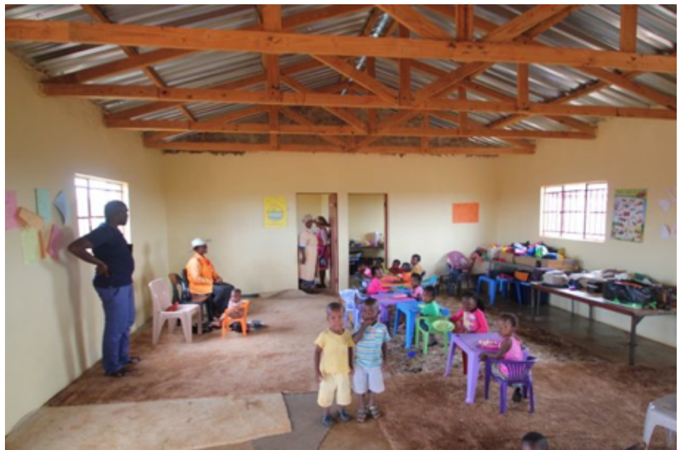
Before: Crèche prior to the installation of the ceiling, which was very cold in the winter and hot in the summer. They also had no access to electricity (Grace Stead, 2015).
