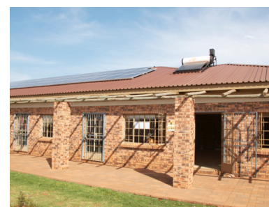
Solar water heater and solar PV array on the roof of the Doornkop Community Centre to provide electricity for the community centre, crèche and old age day care centre (Grace Stead, 2015)
