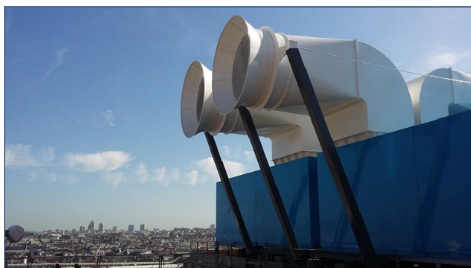
New air-to-air heat pumps on the roof of Centre Pompidou. Photo: Dalkia
