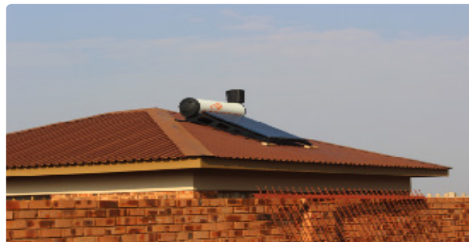
Solar hot water heating system on roof
