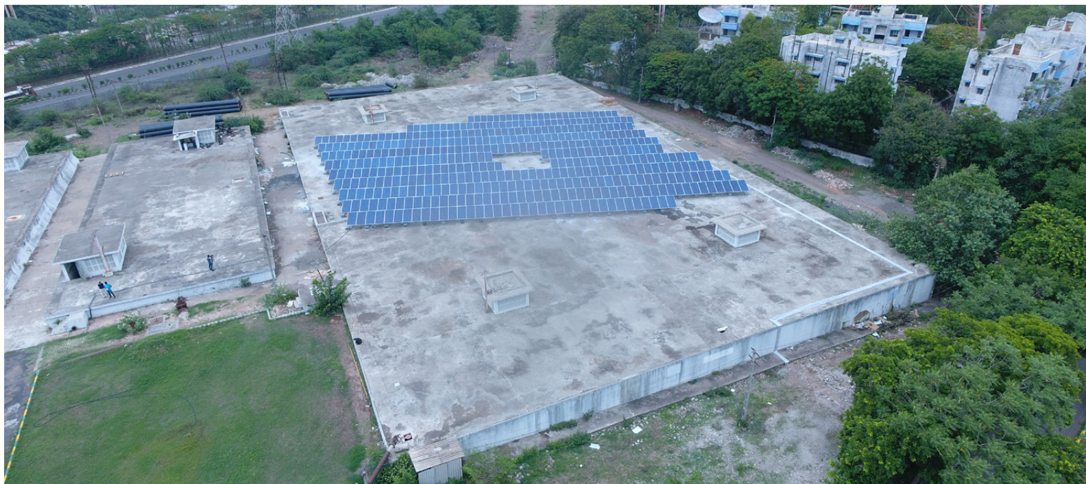
Rajkot, India, and Urban-LEDS project city, has installed a 145kWp solar PV system to help power its Aji water treatment plant
