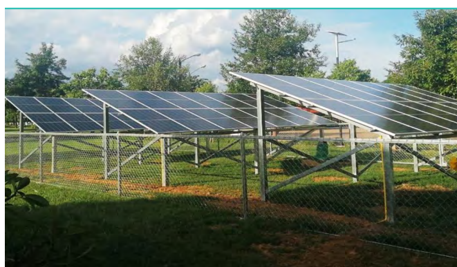
15 kWp Grid-Connected Solar Photovoltaic Systems and solar LED street lights installed at the Nouhak Phoumsavanh Public Park
