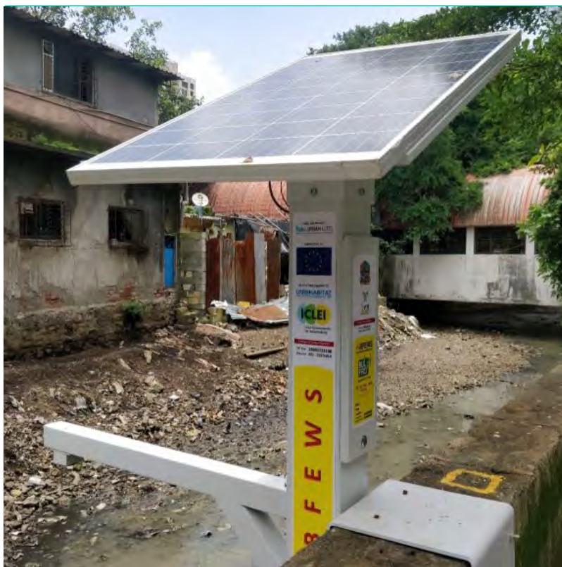
Water level sensor installed at B.N. Bandodkar (Thana) College
